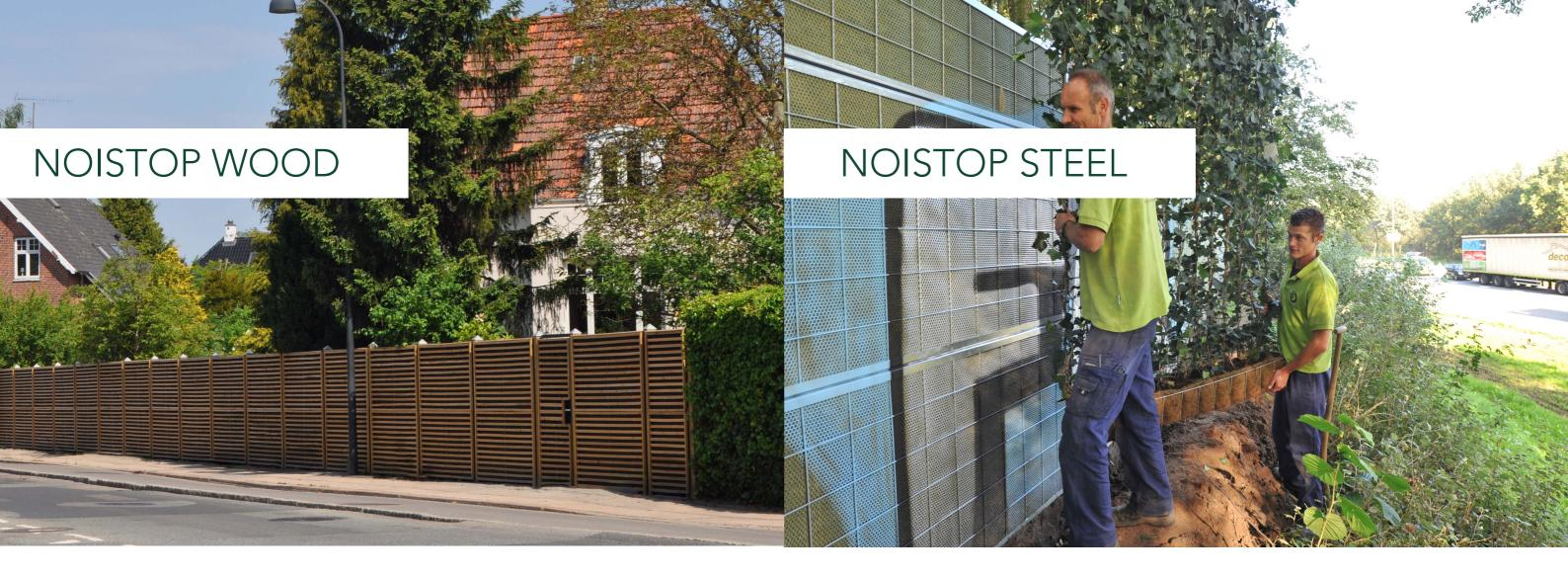
With NoiStop Wood the mineral wool core is wrapped with a black mesh. The mineral wool is sandwiched between aluminium strips with impregnated wooden slats attached. The screens are easy to customise to a fixed size. For NoiStop Wood, delivery times and conditions are on request.
